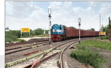
Solapur – Mohol B.G Railway Line
