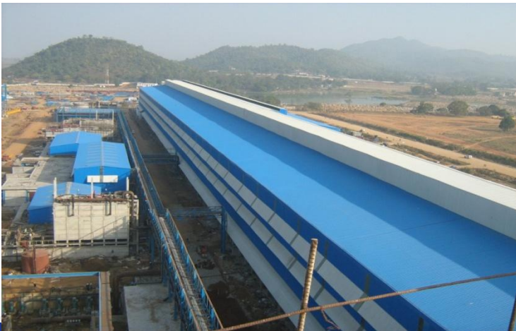
WIRE & BAR MILL PROJECT AT JSPL
