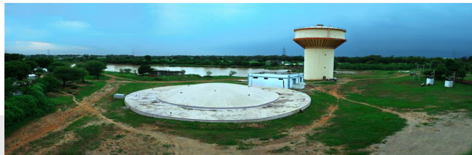
24.86 MLD at Vallibhipur
