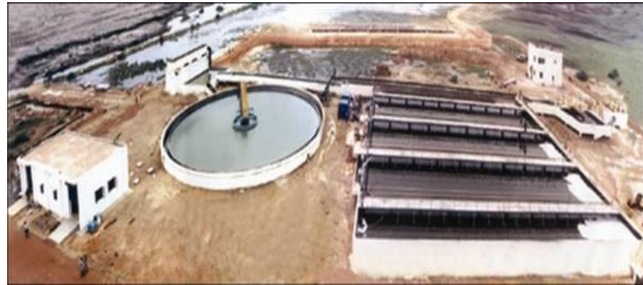
ALANDUR – SEWAGE TREATMENT PLANT
