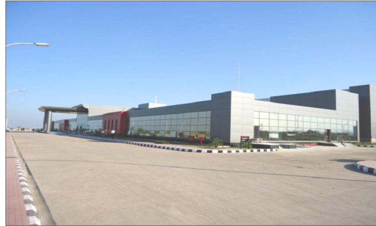
MAIN PLANT BUILDING, TATA CUMMINS
