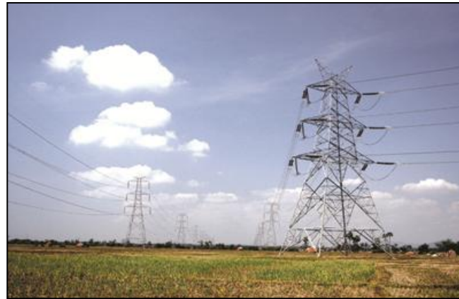
400 KV DC TRANSMISSION LINE PROJECT FOR AP TRANSCO
