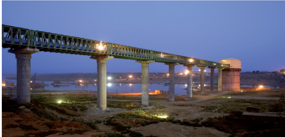
Chambal - Dholpur – Bharatpur Water Supply Project, Rajasthan
