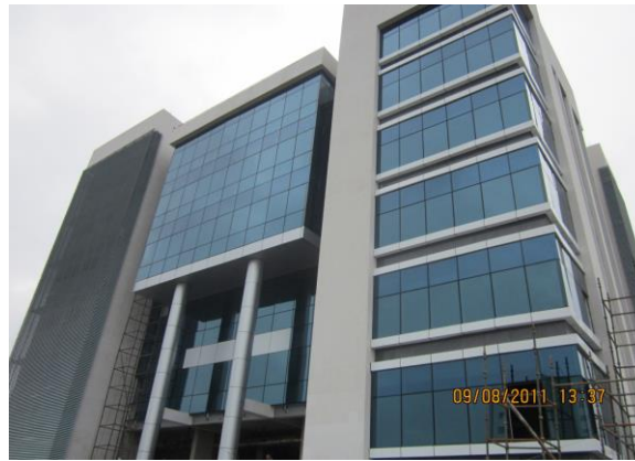
HPCL Administrative Building Kolkata
