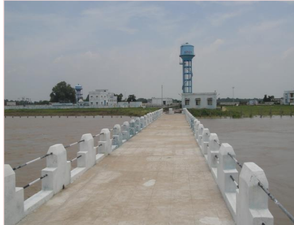
Rural Pipes Water Supply, Bhojpur Arrah Bihar
