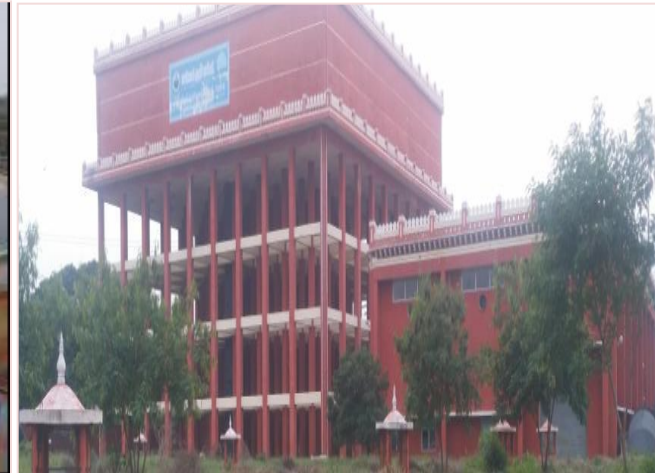
Kilpauk Water Distribution Project Tamil Nadu
