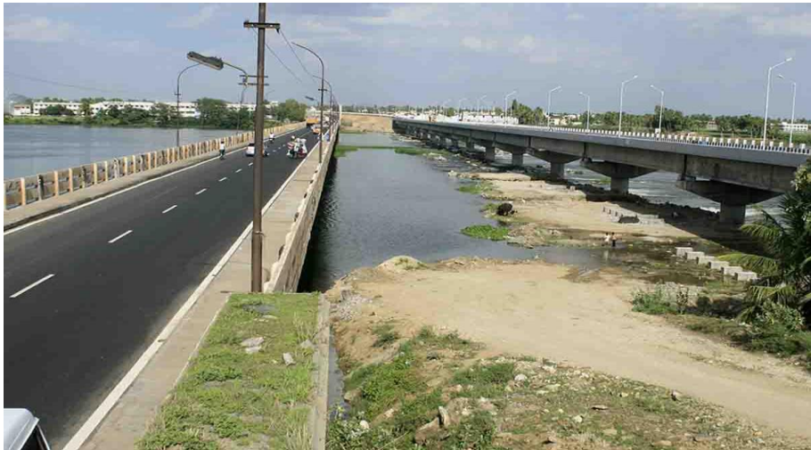
Major Bridge across Caurvey River
