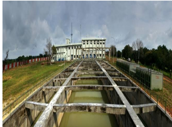
Make-up Water System Package for Super Thermal Power Project, Stage - I (3x660 MW) at Sipat
