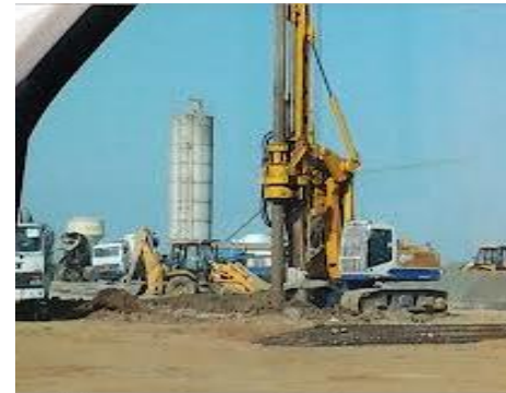
Piling: 3.43 lac meters (500 mm -1600 mm)
