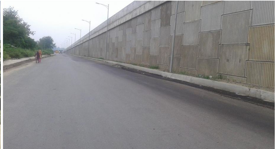
RE Wall Work Jalandhar Amritsar Highway Project
