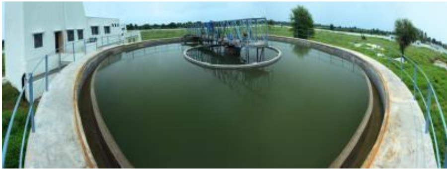
160 MLD Hogenakkal Project, Tamil Nadu
