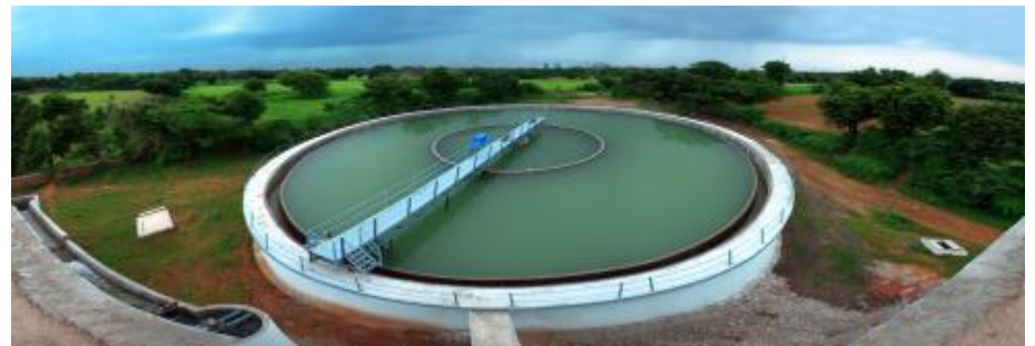
33.24 MLD at Gadhadra
