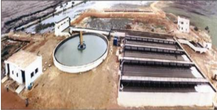
Alandur – Sewage Treatment Plant (12 MLD)
