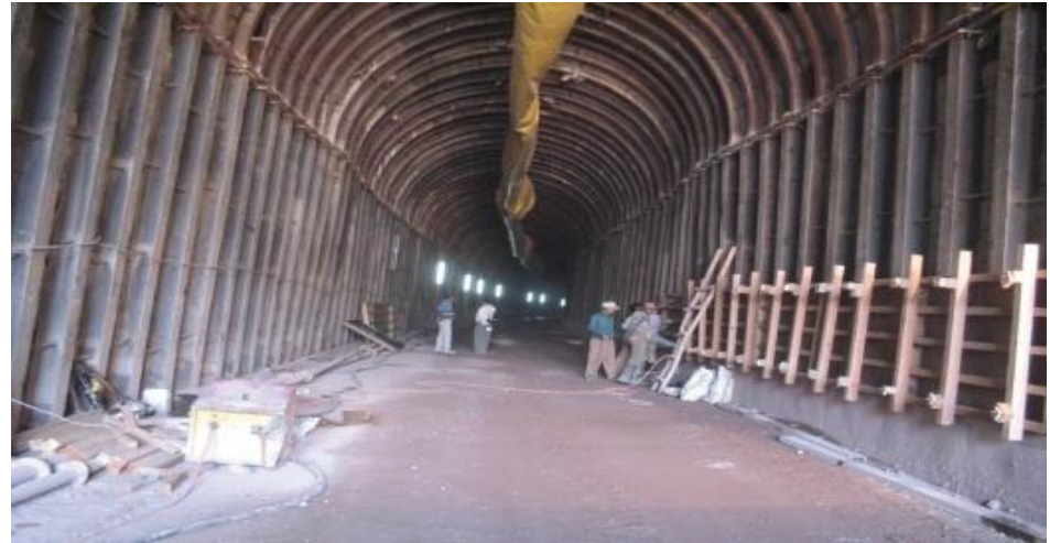
J&K Railway Tunnel
