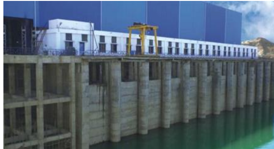
Sripada Sagar lift Irrigation Scheme
