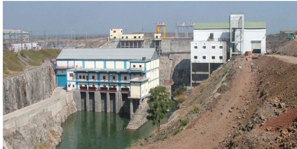
Punasa Lift Irrigation Scheme
