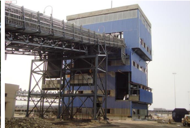
External Coal Handling System (ECHS) Gujarat
