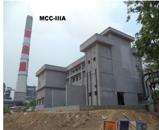
Coal Handling Plant for NTPC Rihand STPP
