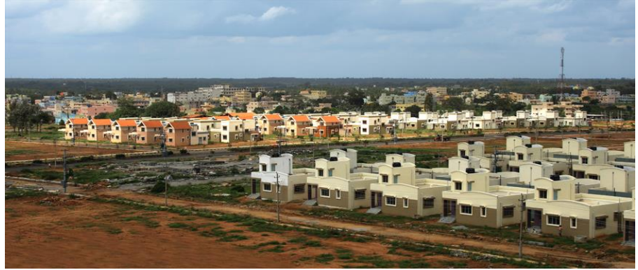
Banahalli Housing Colony - Karnataka
