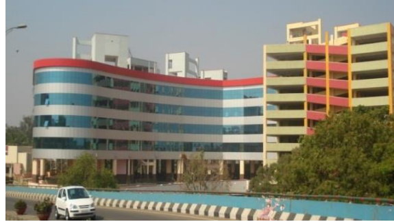
Traffic & Transit Mgmt Center for BMTC at Bangalore
