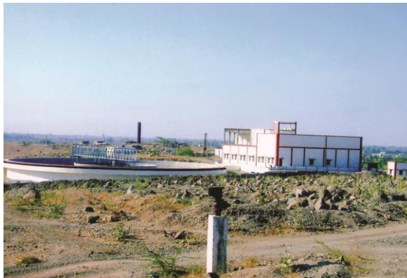
Water Supply Scheme at Cherthala Kerala
