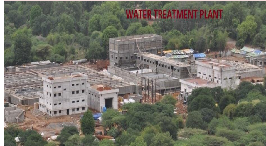
Hogenakkal Water Supply and Fluorosis Mitigation Project, Tamil Nadu
