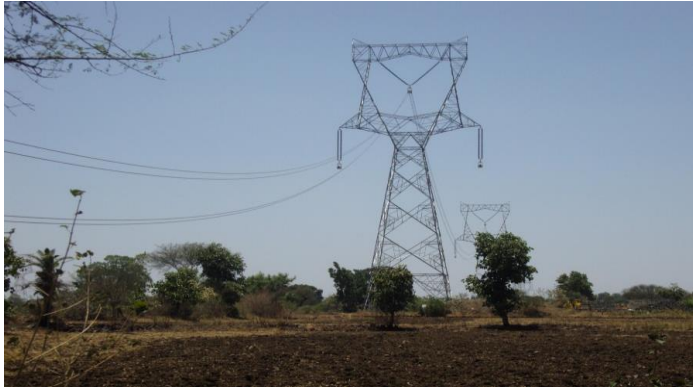
765 KV S/C Transmission Line Angul PS - Jharsuguda PS for PGCIL
