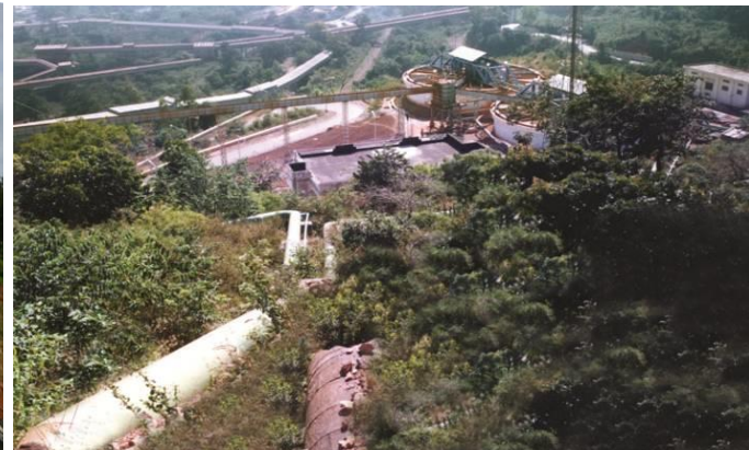
Bailadilla Iron Ore Water Supply Project - NMDC
