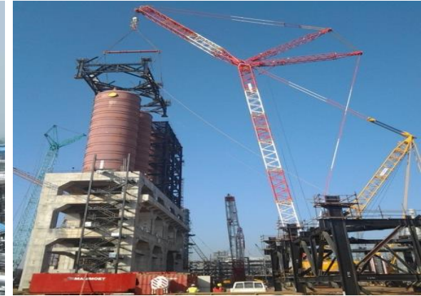
Coke Drum Area of Delayed Coker Unit of Paradip Refinery Project for IOCL
