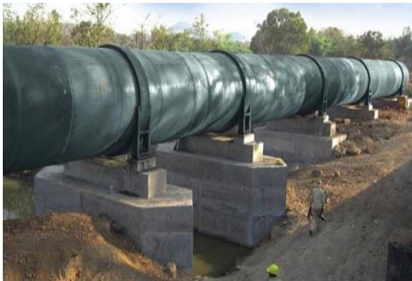
Tansa Transmission Main Pipeline Project Maharashtra
