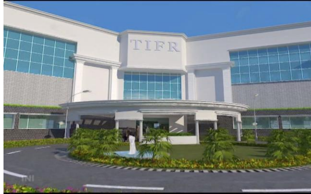
Research & Technical Building for TIFR - Hyderabad
