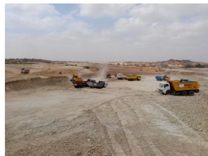
Bura Canal work in progress
