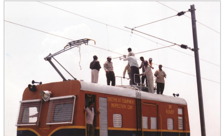
Traction (25 KV AC) OHE works: 60 Track km
