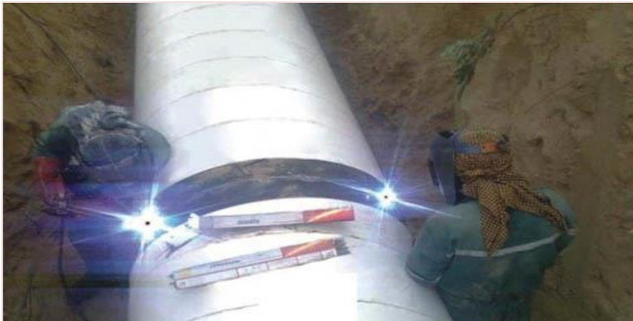
Narmada Water Supply Scheme, Gujarat
