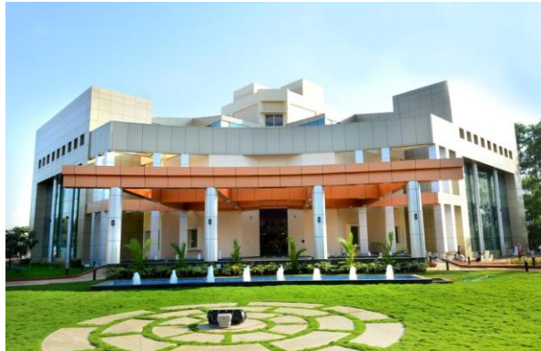
Offsite Building Phase –III Mangalore Refinery & Petrochemical Ltd at Mangalore - Karnataka
