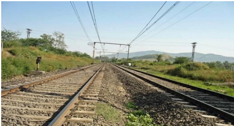
Railway Track Works of 75 km
