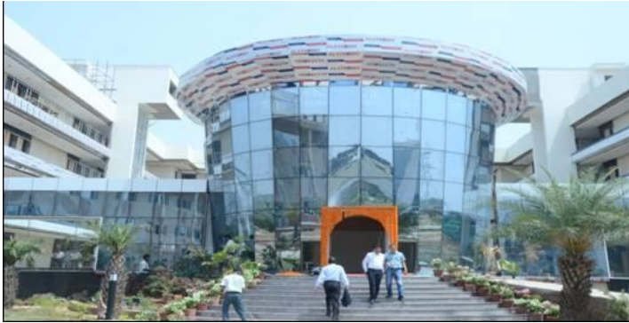
National Transmission & Asset Management Centre (NTAMC) & NPTMC Centre & Trainees Hostel for PGCIL - Haryana
