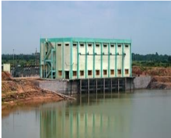
Sardar Sarovar (Narmada) Project, Pumping Station Gujarat
