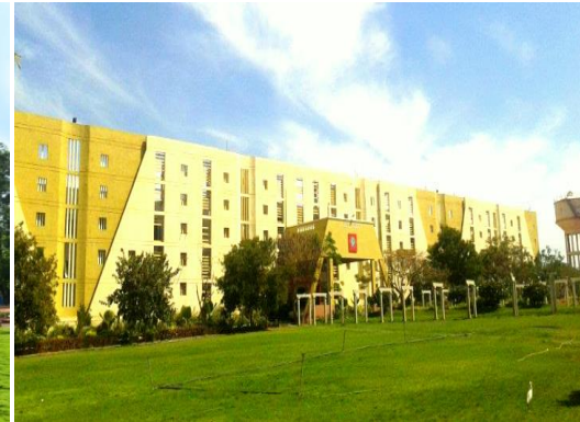
Administrative Bldg Vavodaya Institute of Technology, Raichur – Karnataka
