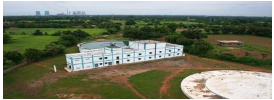
112 MLD Chambal - Dholpur - Bharatpur Project, Rajasthan
