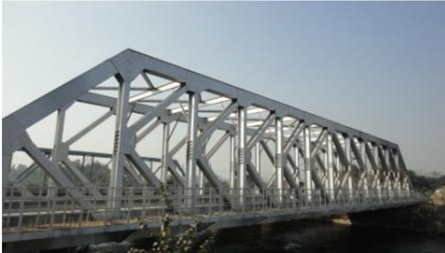
Steel bridge Bhogpur - Mukerian Section
