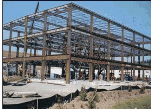
60,600 MT of Structural Steel
